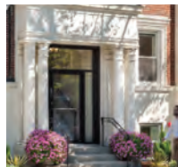
2 Charles Chauncy 1 & 3 Chauncy Street
