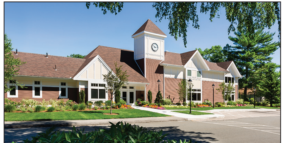
Village Green Apartments clubhouse (after renovation)
