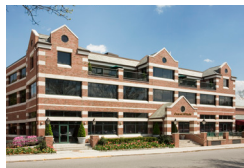
CHR builds headquarters at 300 Independence Drive, Chestnut Hill
